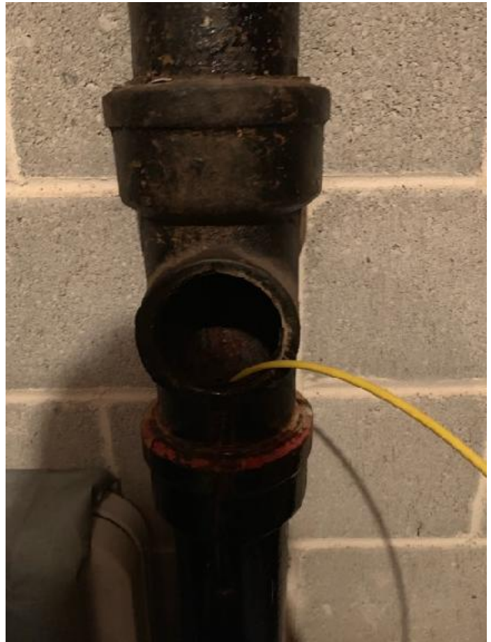
IMAGE OF CAMERA INSERTED INTO SEWER LINE:
