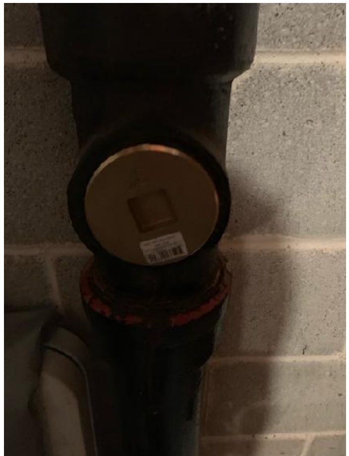
IMAGE OF CLEANOUT AFTER INSPECTION COMPLETION:
